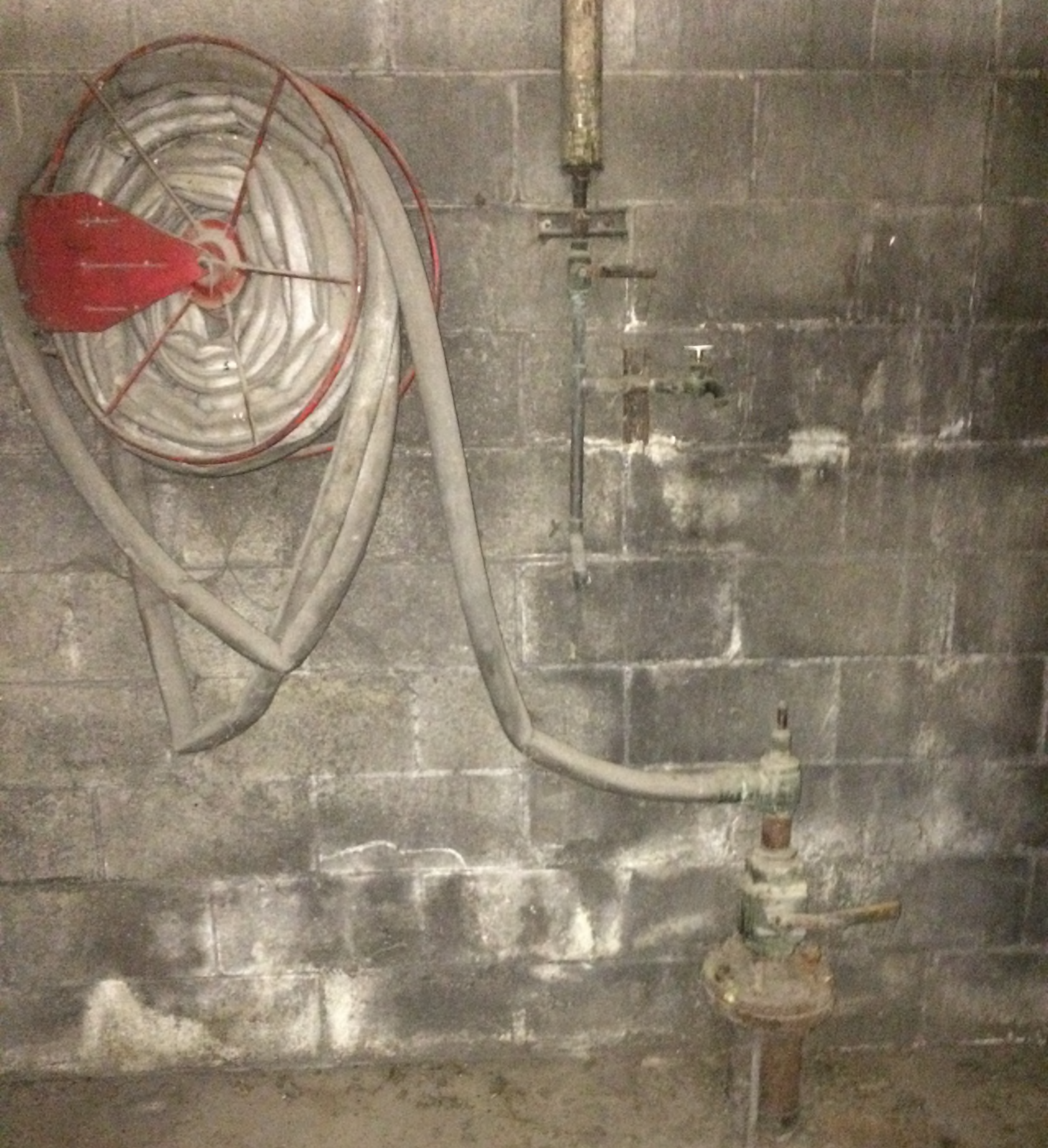
Fire hose station located on northwest wall in central section of building
